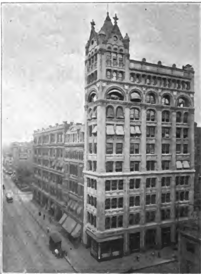
SHERMAN BANK, BROADWAY, NORTHEAST CORNER OF 18TH STREET.
